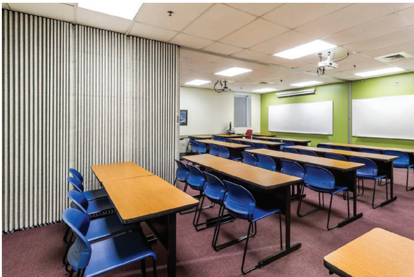
STC 31 test performed by Riverbank Acoustical Laboratories, Geneva, IL. ASTM designation E90-86T
