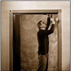
Transfer the door to the attached end of the track. Finish attaching the track with  $1\frac{1}{2}$ " #8 Pan Head screws.
