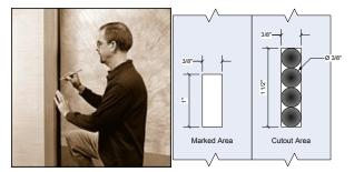
Trace the  $\frac{3}{2}$ " x 1" slot in the Interlocking Jamb Molding onto the wall. Remove the Interlocking Jam Molding and add  $\frac{1}{2}$ " to the top of the tracing.
